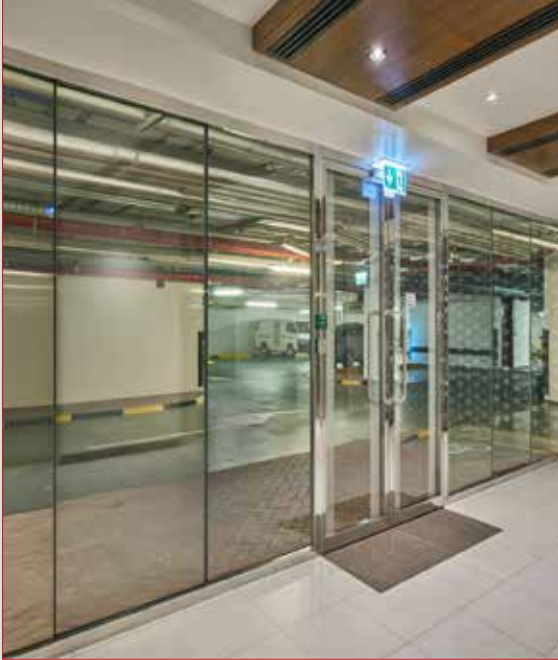
Fully Glazed Butt Joint System - Integrity and Insulation
