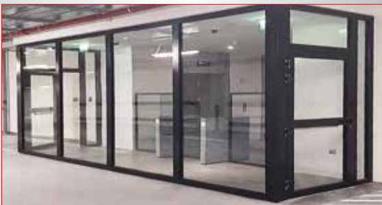
Fully Glazed Butt Joint System - Integrity and Insulation
