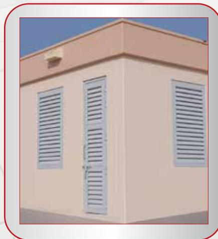
**Fully Louvered Doors (Substation Sand Trap Doors)**
