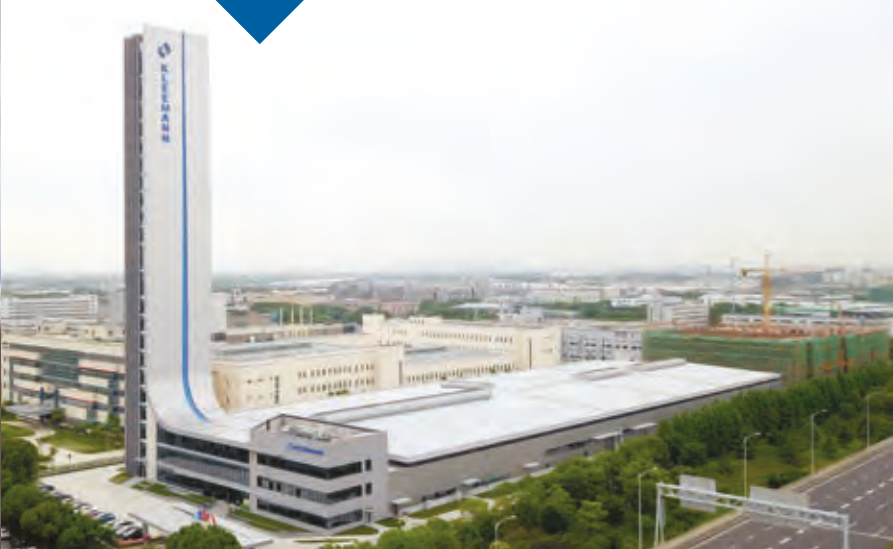
KLEEMANN China testing tower
